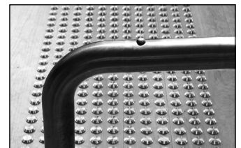
HANDRAIL TACTILE INDICATORS
