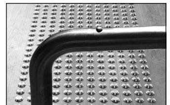
HANDRAIL TACTILE INDICATORS
