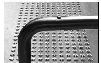
HANDRAIL TACTILE INDICATORS
